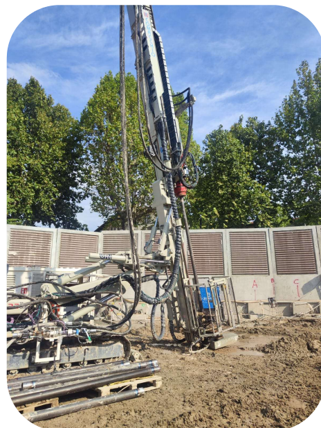
Area 1 estesa Jet grouting
